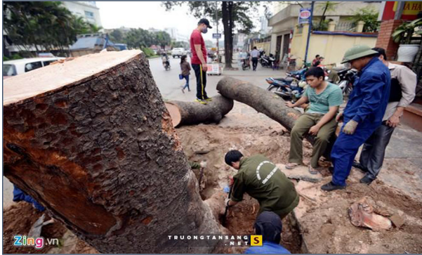
Fig. 1 Healthy old trees were chopped down. Hanoi looked like a construction site. Source http://www.doisongphapluat.com . Available at http://www.doisongphapluat.com/xa-hoi/ha-noi-chat-6700-cay-xanh-gs-ngo-bao-chau-len-tieng-a87881.html
