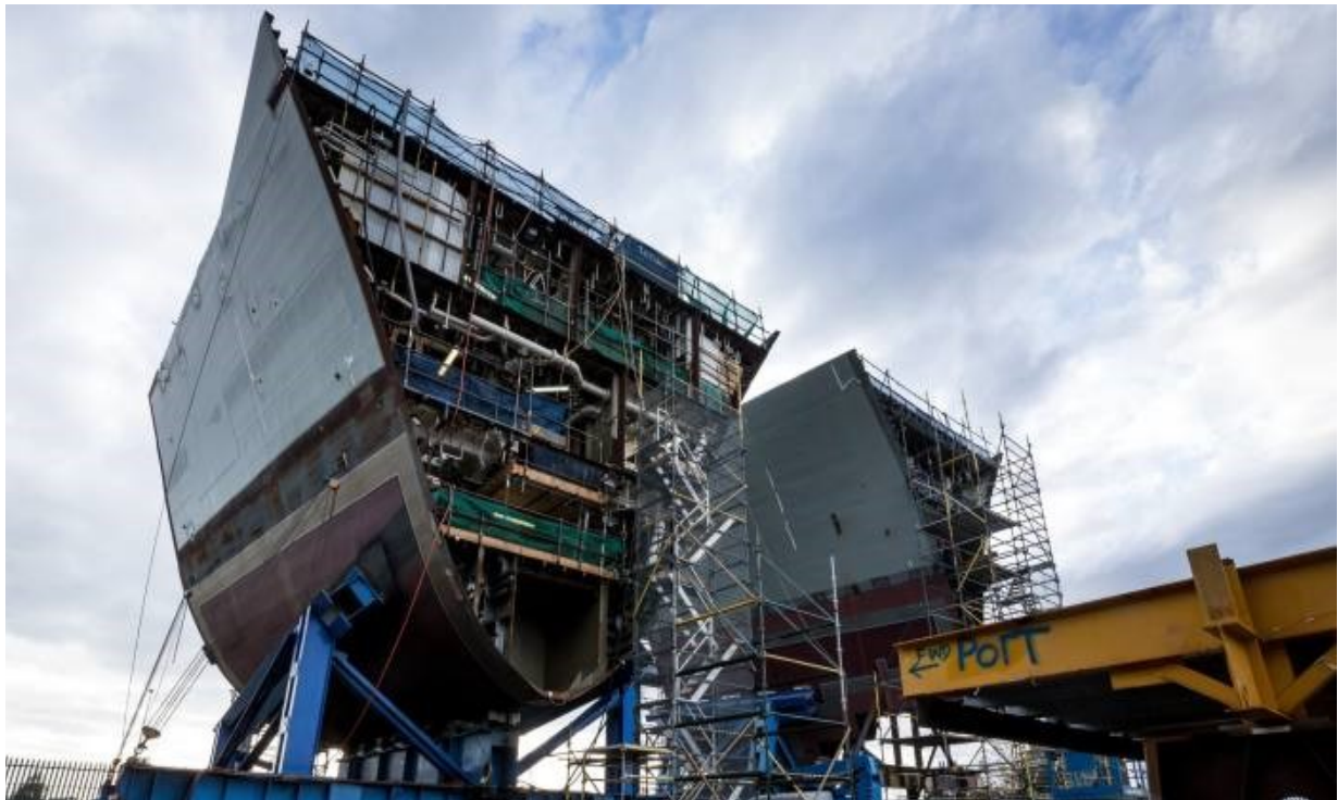
HMAS Sydney, an air warfare destroyer, under construction in Adelaide © Bloomberg
